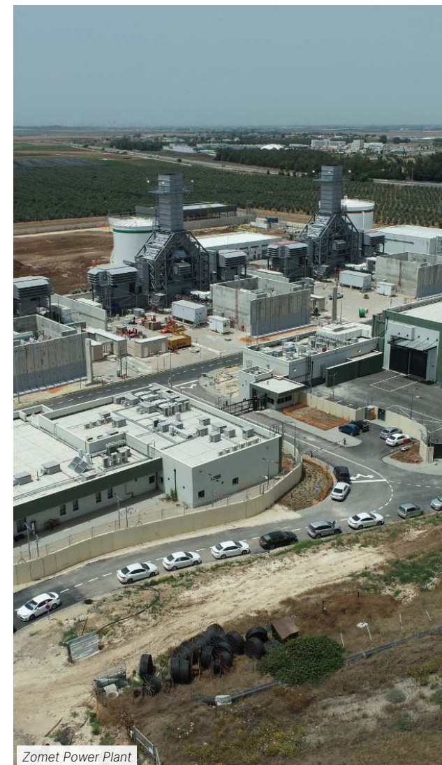
Zomet Power Plant
