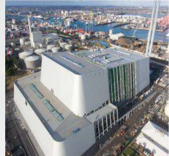
Dublin, Ireland Covanta Energy
